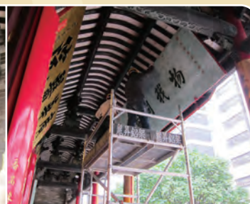
拆卸千步廊的牌匾對聯以作修復 Dismantling of the plaques and couplets at the verandah for conservation
